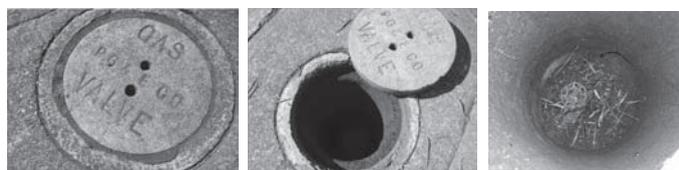
One of these photos shows a valve access "box" with the lid removed. In this case the valve was clearly visible and could be tested. In the other photo is a lid that has obviously not been lifted off for a very long time. In this latter case, the valve could be covered by a foot or more of soil and the resulting delay to reach the shut-off could be a problem if a gas leak was detected in the home.
